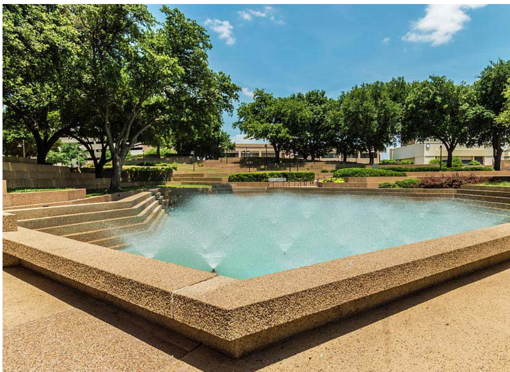
Hồ Sục Khí (Aerated Pool)
